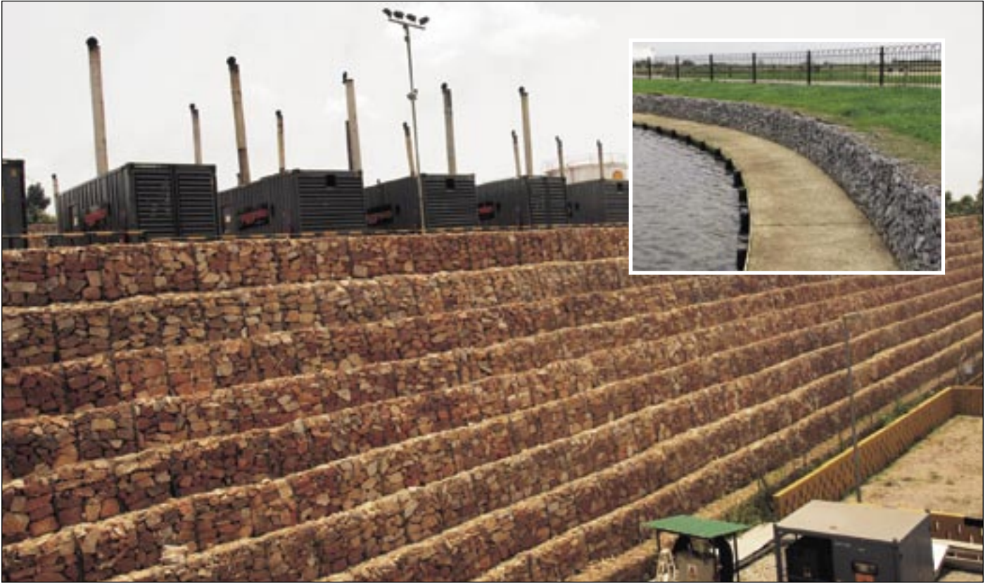
▲ 10m high mass gravity woven wire gabion wall designed and constructed in Kampala, Uganda.
