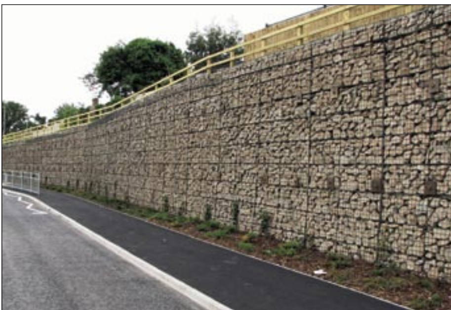
▲ Gabion cladding to steel sheet piles at Dovercourt, Essex.
