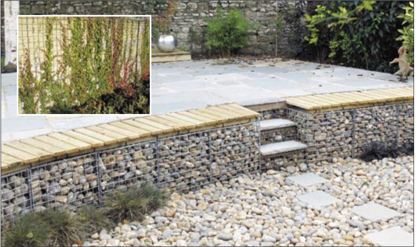
▲ A typical landscape example, where smaller mesh apertures have been utilised to contain a rounded stone fill to achieve the desired aesthetic effect.
