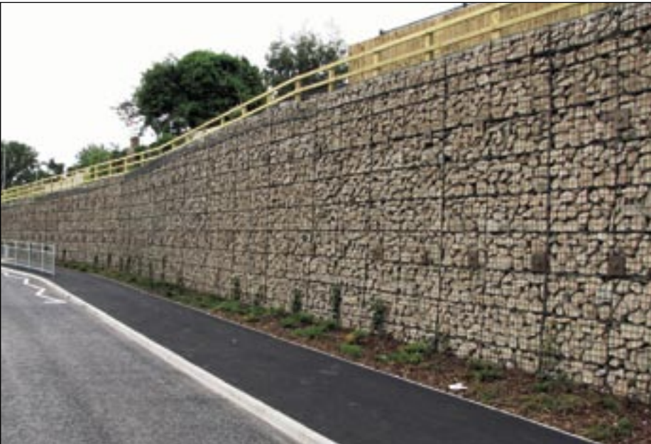
▲ Gabion cladding to steel sheet piles at Dovercourt, Essex.
