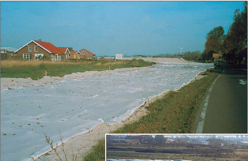
reinforcement with Stabilenka®150/45 for the access to the Jever bypass, Germany
