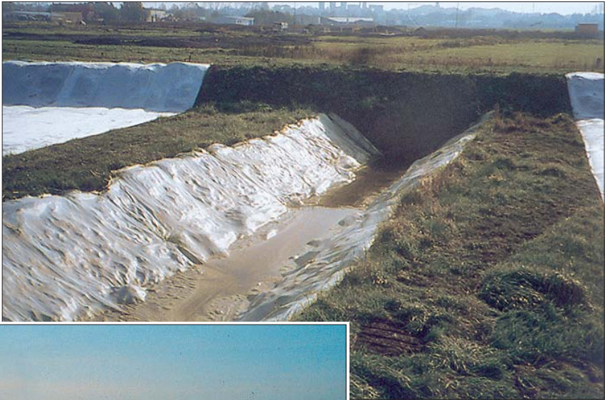
additional reinforcement to existing trenches
