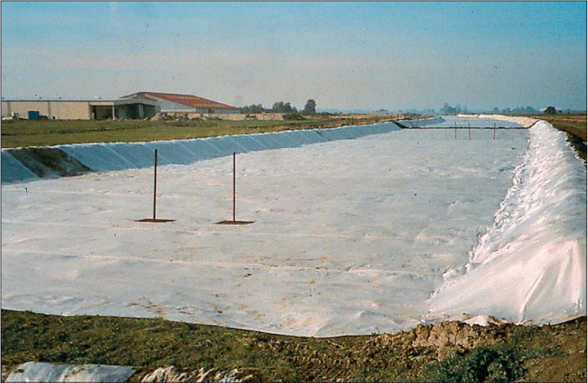
reinforcement with Stabilenka® 300/45 for the bypass embankment
